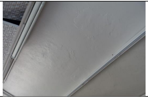
Figure 56 – Damp damage to plaster ceiling over stage in function room. (Source NBRSArchitecture, March 2018)
