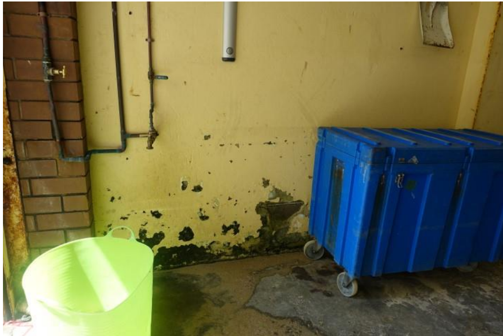
Figure 73 – Damp damage to walls in boat shed. (Source NBRSArchitecture, March 2018)
