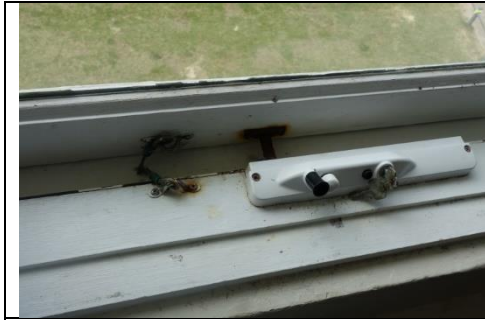
Figure 63 – Corrosion to window winders on second floor. (Source NBRSArchitecture, March 2018)
