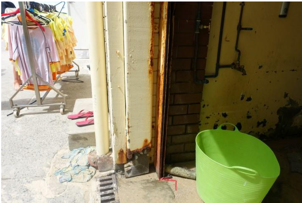
Figure 72 – Corroded door frame to boat shed. (Source NBRSArchitecture, March 2018)
