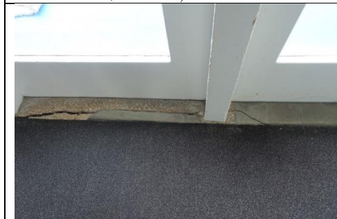
Figure 57 – Cracking in terrazzo door sill to balcony on first floor. (Source NBRSArchitecture, March 2018)
